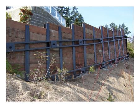
This is a small soldier pile wall with tie backs. The vertical elements are the "soldier piles" spaced about 6 feet on center here. They are steel "H" sections weighing 30 lbs per foot. The two rows of horizontal elements are whalers. Between every other soldier pile notice the square plate with the road sticking out of it. These rods extend into the soil about 20 feet.
