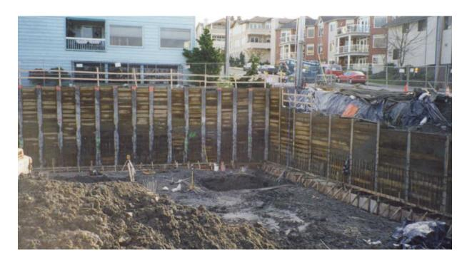
This is a cantilevered soldier pile wall. It does not use tiebacks. Often tiebacks cannot be used because the walls are on or near the property line and the tiebacks would extend beyond the property line. The wall in the back is about 16 feet high. The soldier piles are spaced 6' on center and weigh about 120 lbs per foot. the higher the wall the heavier the steel sections need to be.
