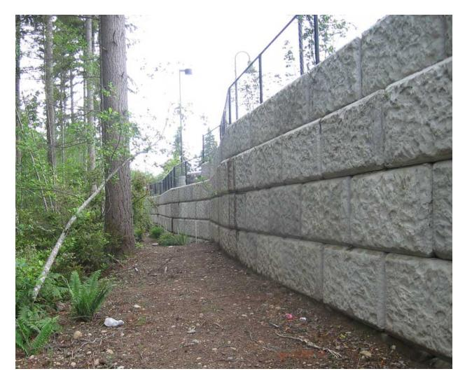
This is one of a class of walls that uses precast concrete elements generically referred to as Mechanically Stabilized Earth (MSE) walls. These walls typically use a geogrid reinforcing matt that ties to each block and extends back into the earth 10 or 15 feet. This wall is about the height we would need at Copalis (8 to 10 feet).
