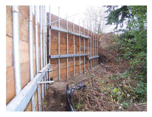
This wall is similar to the soldier pile wall except it uses small diameter "pin" piles spaced at 4 feet on center. It still uses tie backs and whalers. Styrofoam "fill" was used behind the wall to reduce the horizontal force of the soil on the pin piles.
